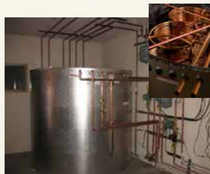
Open Storage Using Immersed Copper Coils for Heat Exchange
