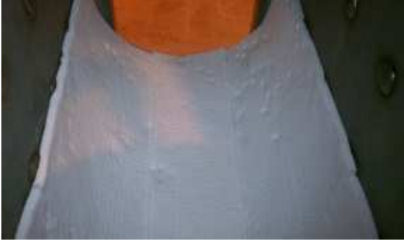
New Ceramic Blanket in Place
