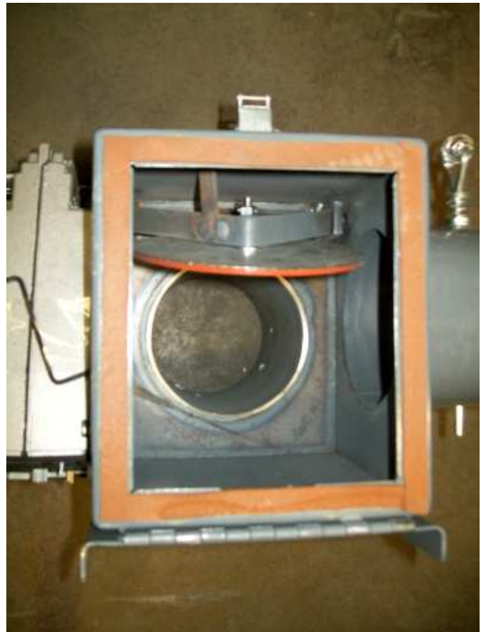
Air Valve Disk in Open Positioning
