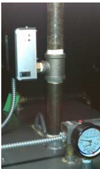
Photo: Low Water Cutoff Installation
