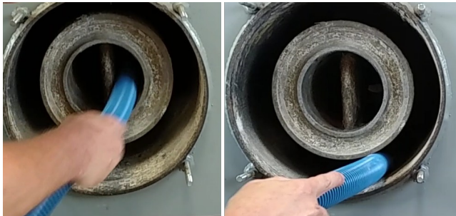
Vacuuming Heat Exchanger
