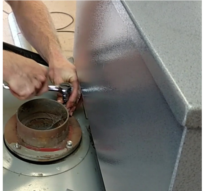
Flue Tube Assembly Bolted Flange
