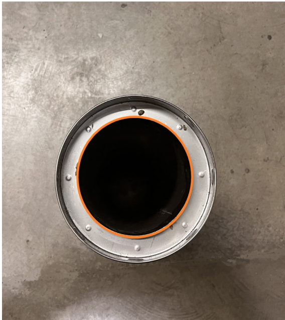
Single Wall to Insulated Stovepipe Connection
