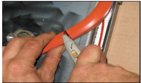
Trimming Preformed Silicone Bead
