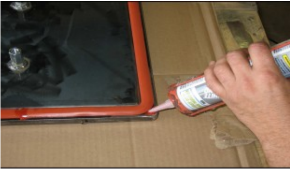
Reinforcing Corners with High Temperature Silicone
