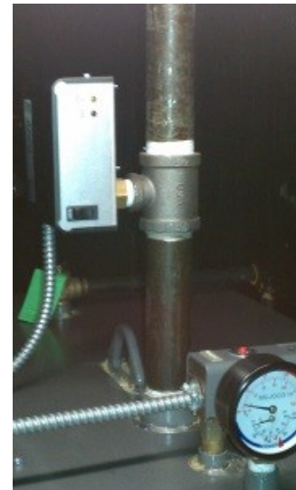
Photo: Low Water Cutoff Installation
