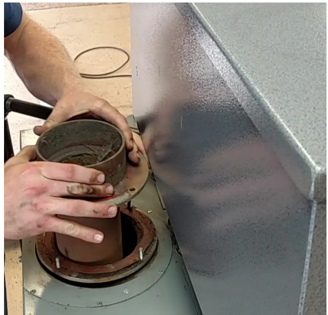
Lifting Out the Flue Tube Assembly
