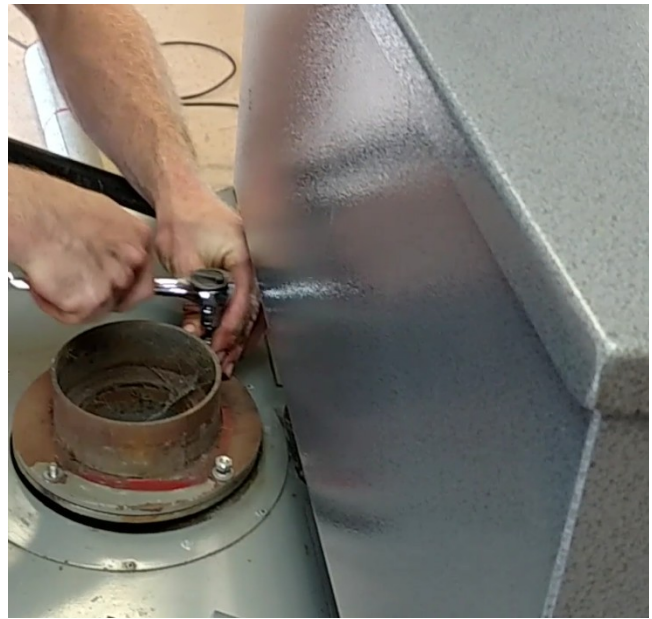
Flue Tube Assembly Bolted Flange
