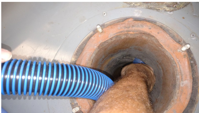
Hose Inserted into Swirl Tube Heat Exchanger
