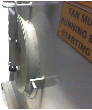
Sight Tube Flap in Closed Position
