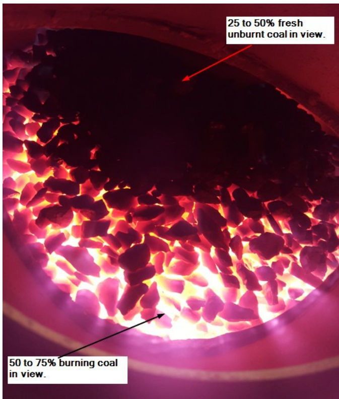
Coal Gun Fire Position
