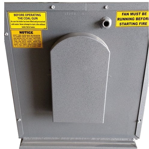
Sight Tube Cover in Place
