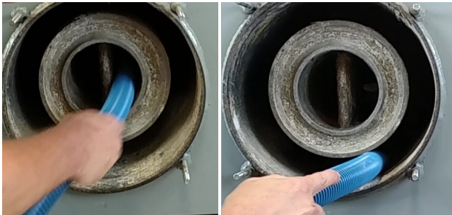
Vacuuming Heat Exchanger
