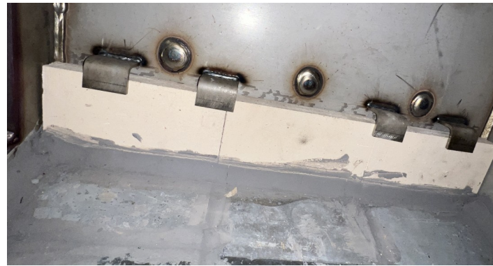
Side-Wall Firebrick Mortored
