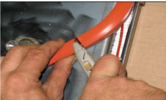
Trimming Preformed Silicone Bead
