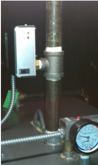
Photo: Low Water Cutoff Installation
