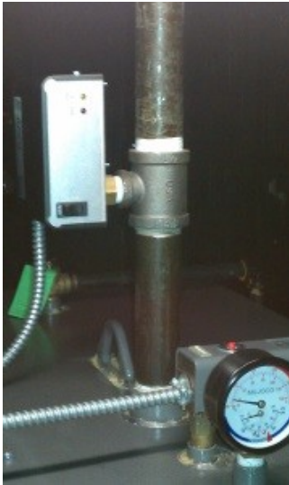
Photo: Low Water Cutoff Installation
