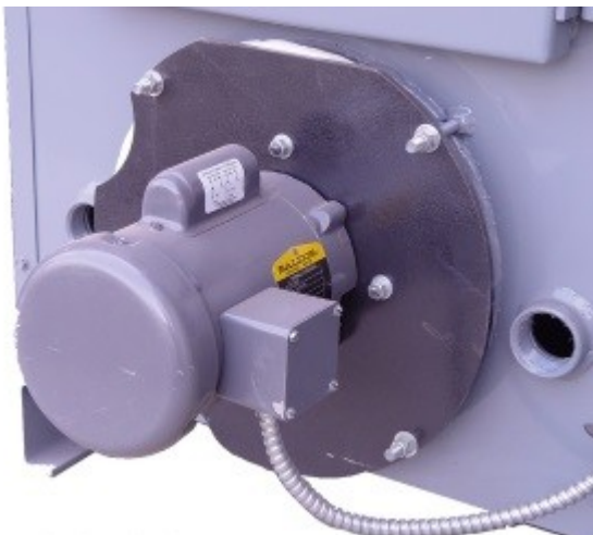
Direct-drive fan attached to boiler
