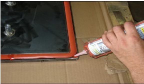
Reinforcing Corners with High Temperature Silicone
