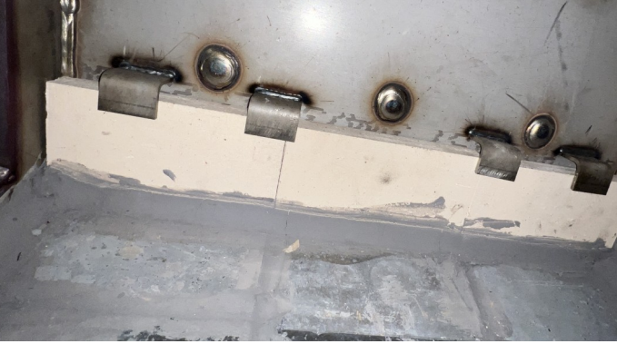
Side-Wall Firebrick Mortored
