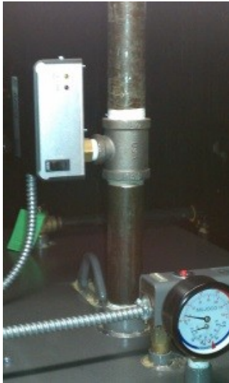
Photo: Low Water Cutoff Installation
