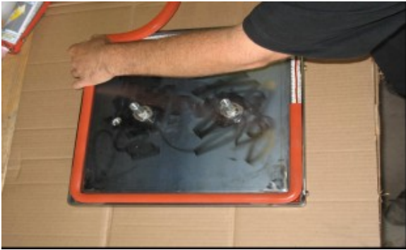
Adding Preformed Silicone Bead to Door
