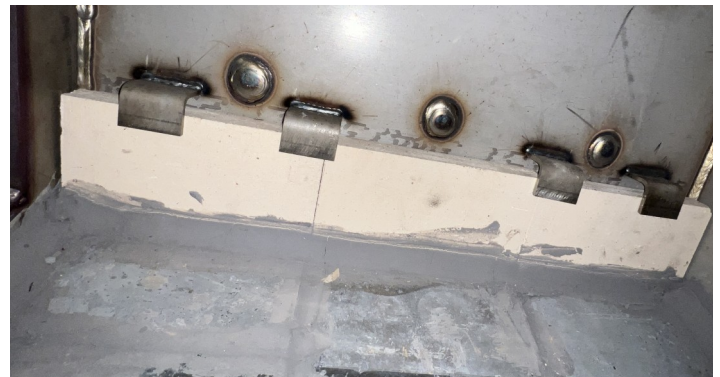
Side-Wall Firebrick Mortored
